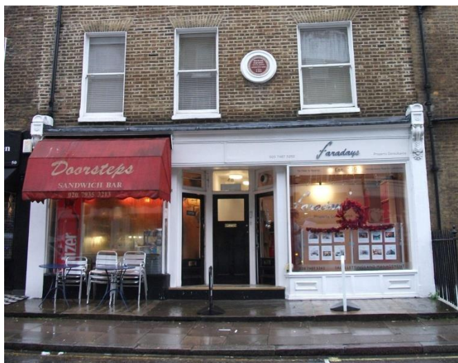
Figure 4: N° 48 Blandford St on 20 December 2012. The house comprises two shops and two apartments, and has three front entrance doors.
