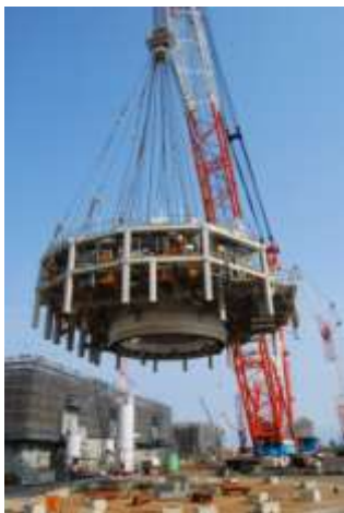
Shimane 3, The Chugoku Electric Power Co., Inc. Source: Hitachi-GE Nuclear Energy, Ltd.
