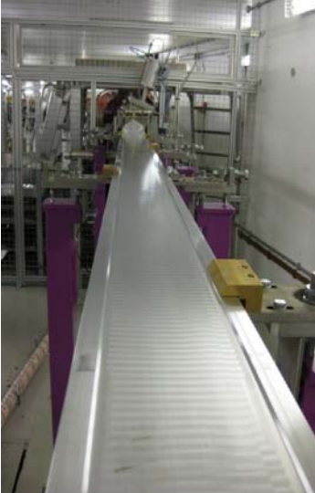
Fig 2: 5 m long extruded aluminium non-evaporable getter (NEG) coated ultra-high vacuum vessel installed at Diamond. The NEG coating pumps active gases such as hydrogen and carbon monoxide and can produce local pressures in the extreme high-vacuum (XHV) range.
