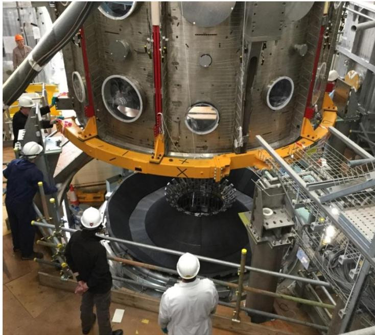
*Image showing the installation of the outer cylinder on to the bottom plate. The super-X divertor tiles can be seen installed on the bottom plate.*
