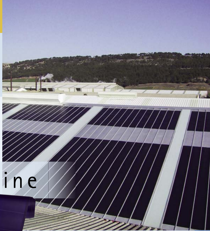
A thin-film amorphous silicon PV array integrated into a roof. Inset: a flexible PV roll United Solar Ovonic
