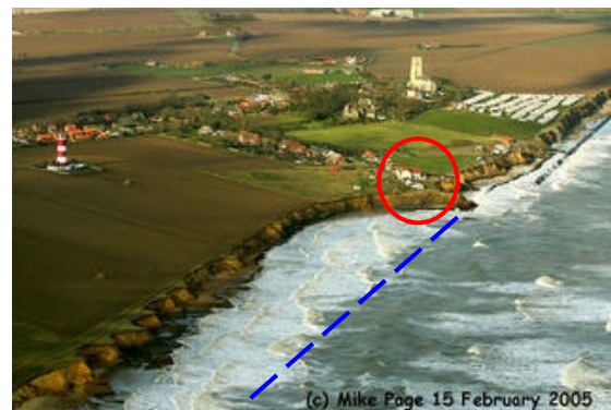
Figure 3 – Coastal erosion forming a bay at Happisburgh, Norfolk. The blue line indicates the position of the cliff before the defences started to fail in 1996. Miss Wrightson's tea shop (circled in red) is dangerously near the cliff edge. Photograph taken by Mike Page, 15 th February 2005. http://www.happisburgh.org.uk/gallery/mikepage
