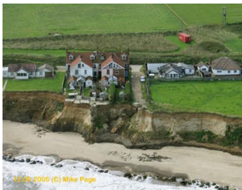
Figure 2 – Miss Wrightson's Cliff House tea shop positioned dangerously near the cliff edge at Happisburgh. Photograph taken by Mike Page, 12 th September 2005. http://www.happisburgh.org.uk/gallery/mikepage
