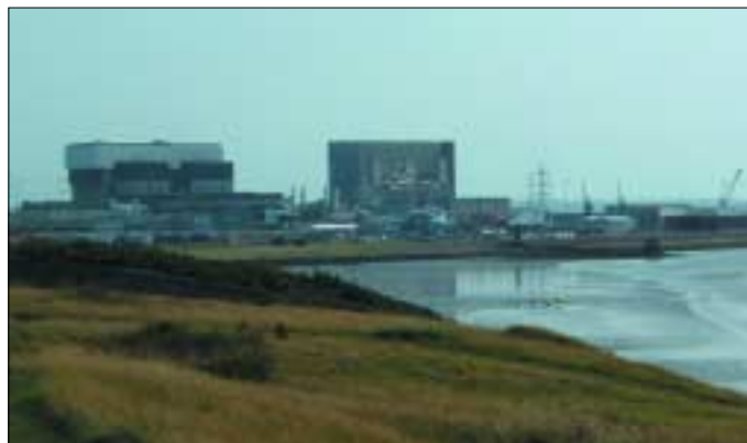
The two nuclear reactors at Heysham, Lancashire, can produce enough electricity to feed a city one-and-a-half times the size of Manchester.
