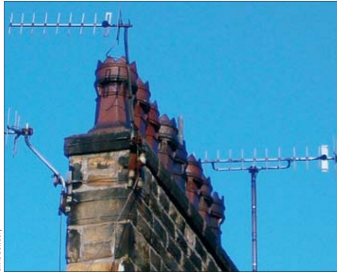
An example of narrowband aerial (top) and a wideband one (right).
